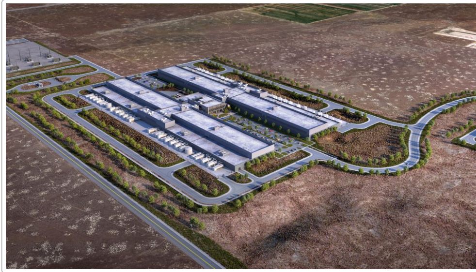
Figure: Rendering of Meta's 960,000 sq ft Kuna data center campus (Meta Platforms). The design includes multiple long data hall buildings (center) and on-site electrical infrastructure (note the dedicated substation yard at left). Such hyperscale facilities were traditionally sized for ~30 MW a decade ago, but today 200 MW campuses are becoming common 9 . Meta's Kuna site is being outfitted as an "AI-ready" data center, with cutting-edge cooling and power systems to handle high-density compute hardware.
